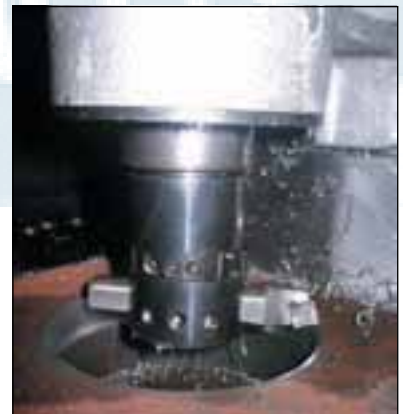
Finishing a drill at a lock gate
